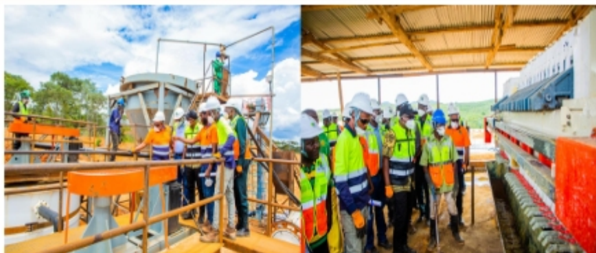
Picha Na. 3: Mheshimiwa Athony P. Mavunde Akikagua Ujenzi wa Kiwanda cha Uongezaji Thamani Madini ya Shaba cha Kampuni ya Mineral Access System Tanzania (MAST).
